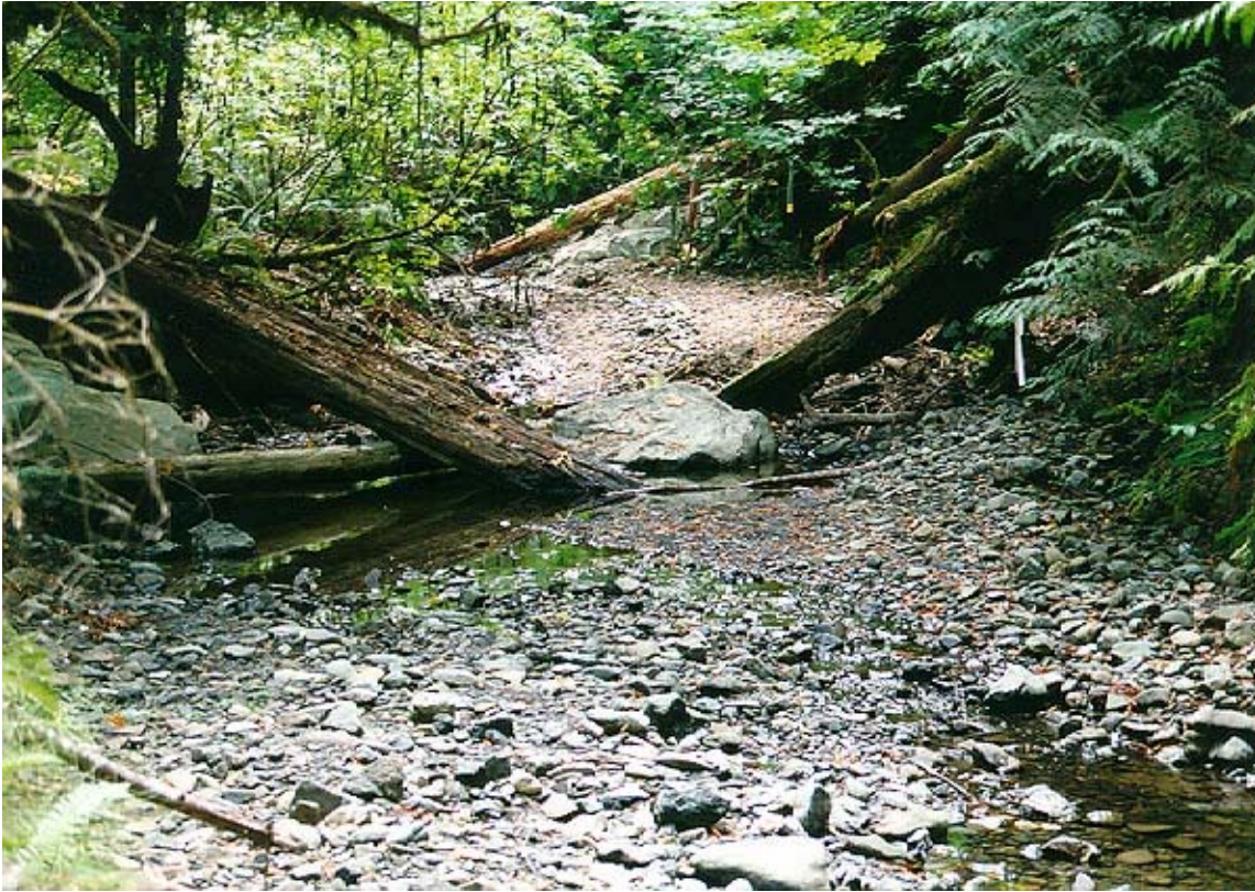
Figure 32. The large wood in the channel of Graham Gulch was installed to help improve sediment routing and pool formation. High bedload transport has caused significant aggradation of the stream that prevents pools from forming. Much of the coarse bedload seen in this photo is coming from the large rotational slump upstream.
